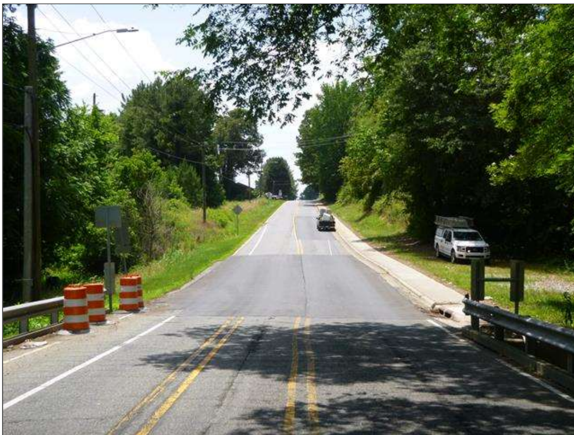
FROM THE DECK, LOOKING SOUTH
