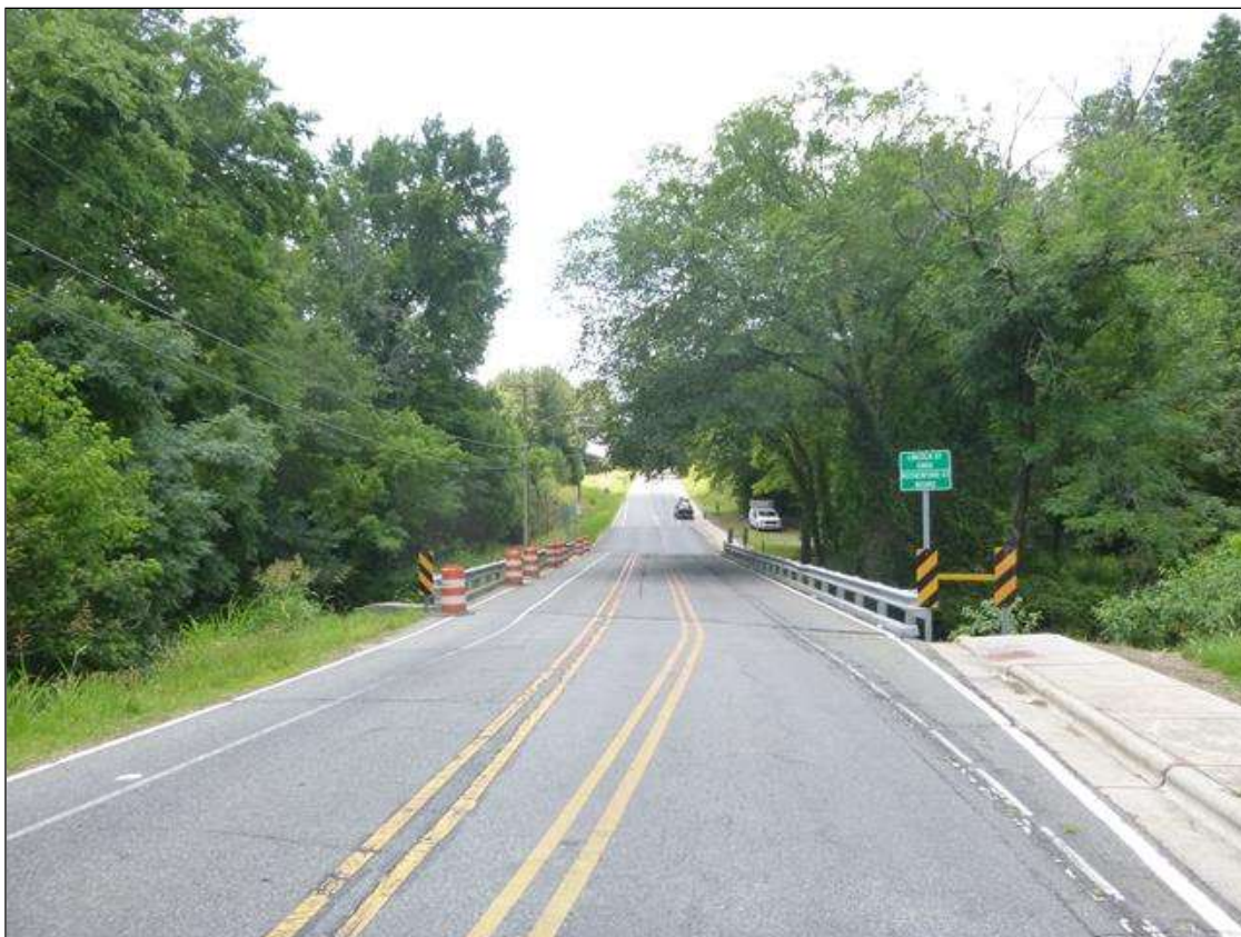
NORTH APPROACH LOOKING SOUTH
