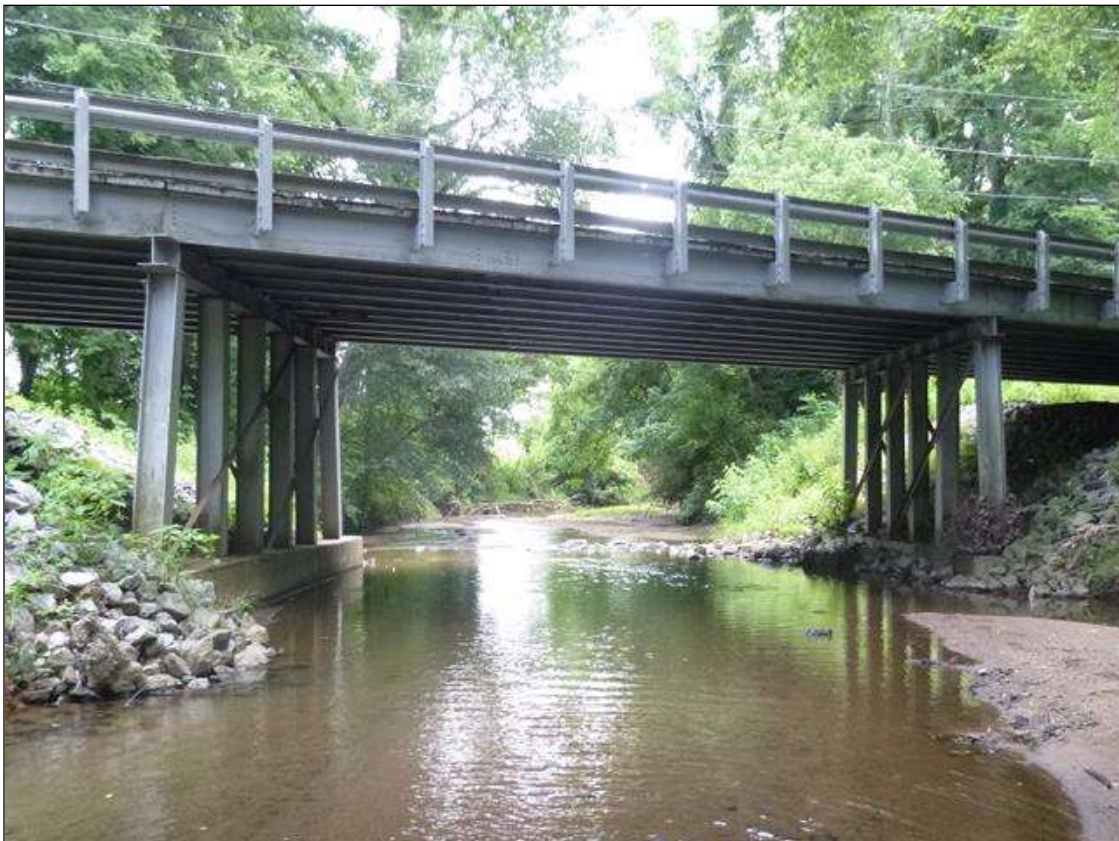
UPSTREAM, LOOKING EAST
