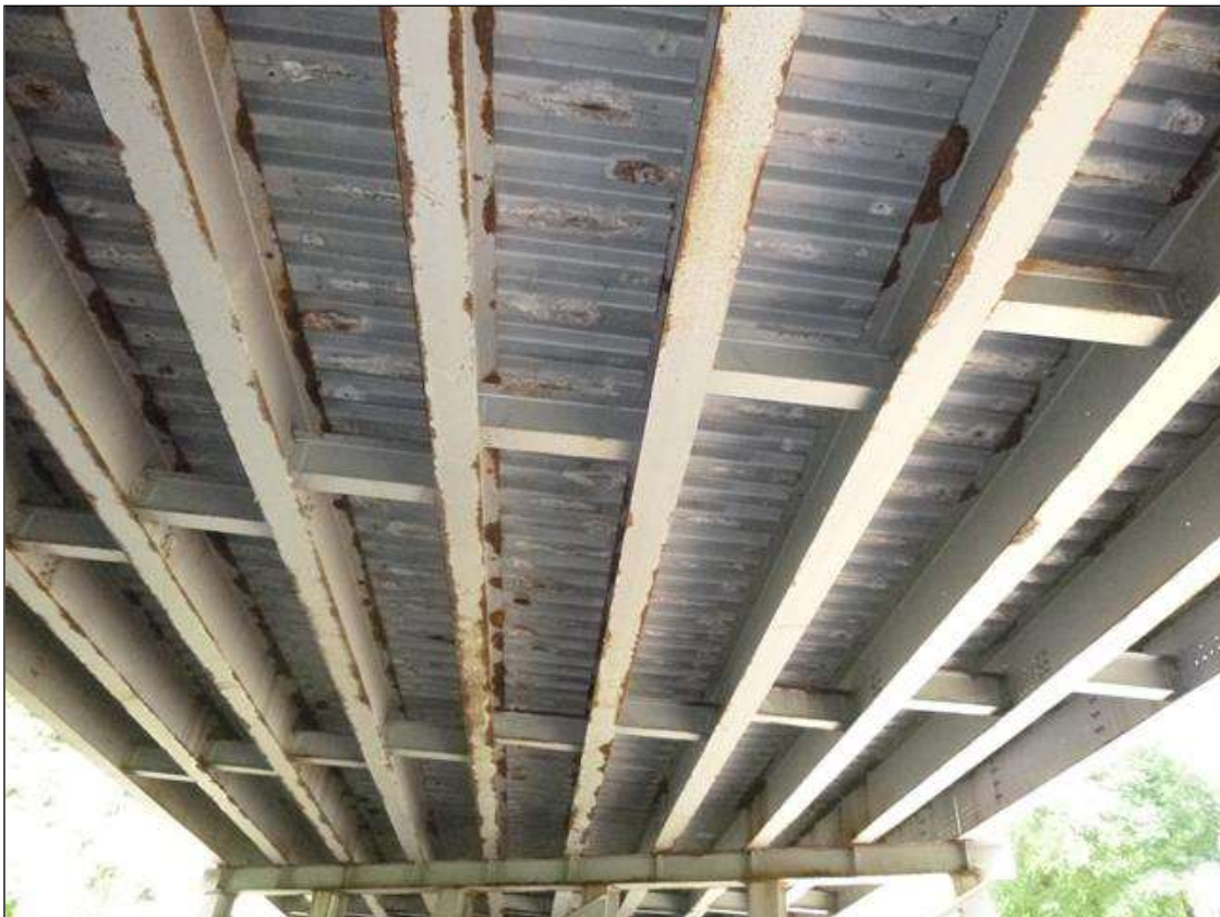
SPAN 2 LOOKING NORTH [ALL SPANS SIMILAR]
