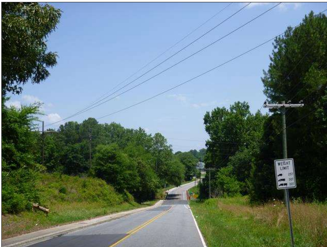
APPROXIMATELY 500' SOUTH OF THE STRUCTURE, POSTING
