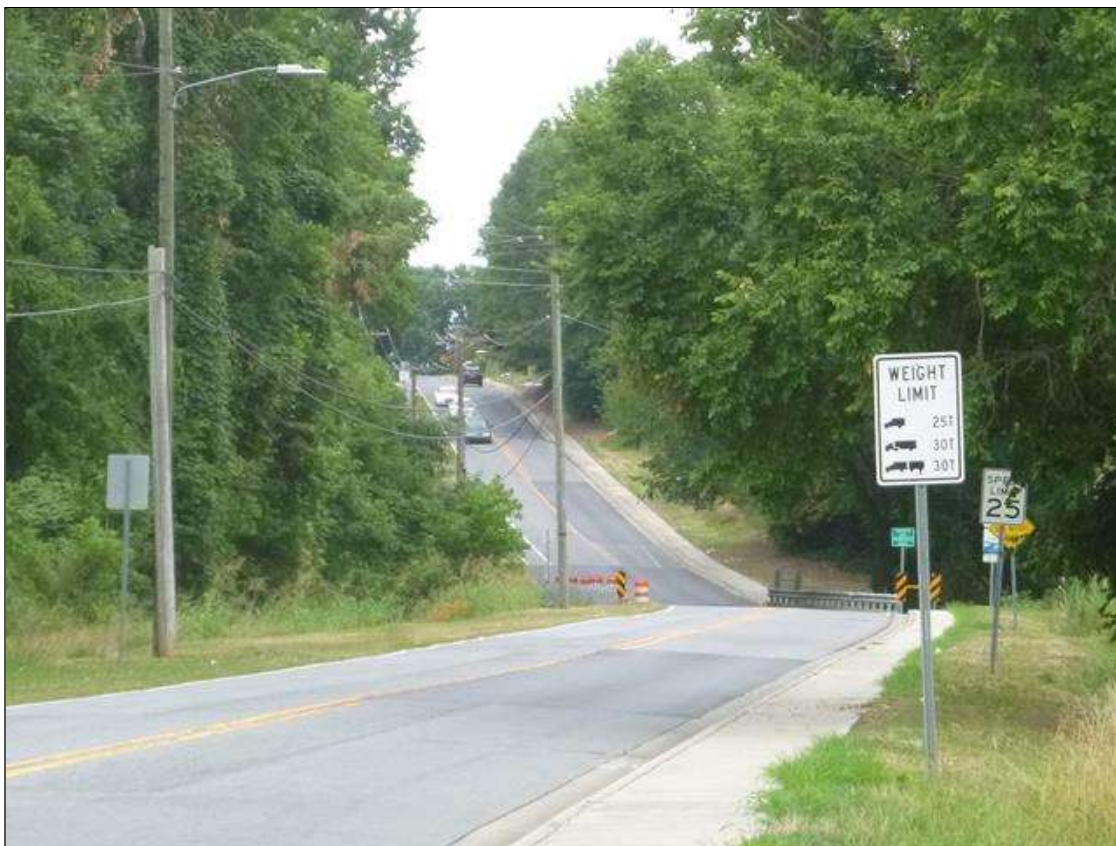
APPROXIMATELY 500' NORTH OF ABUTMENT 2, POSTING
