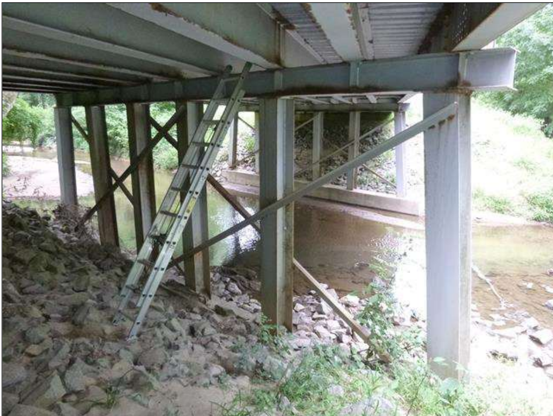
BENT 1 LOOKING NORTH [BENT 2 SIMILAR]
