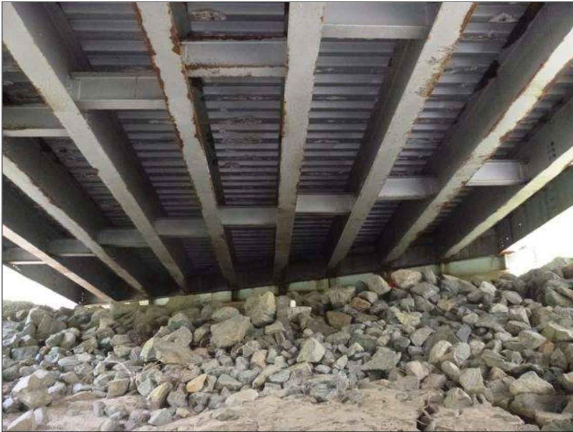
ABUTMENT 2, LOOKING NORTH
