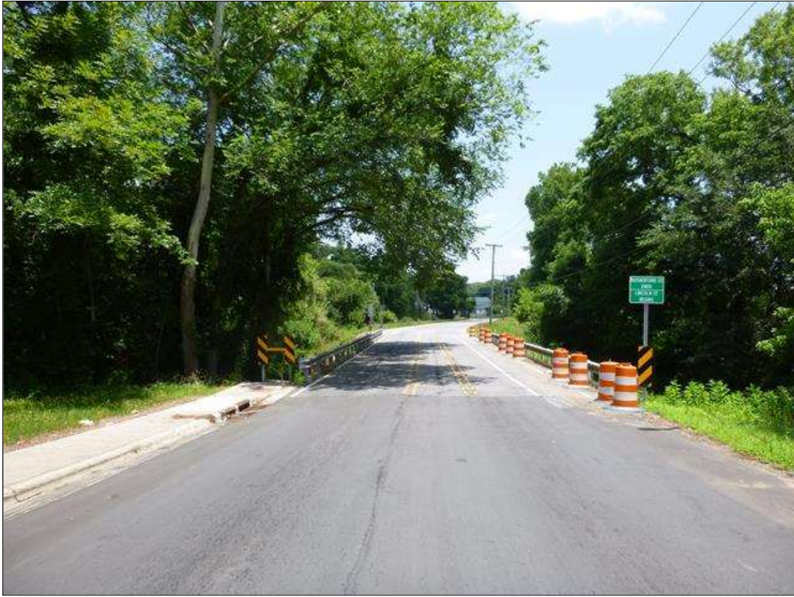
SOUTH APPROACH LOOKING NORTH
