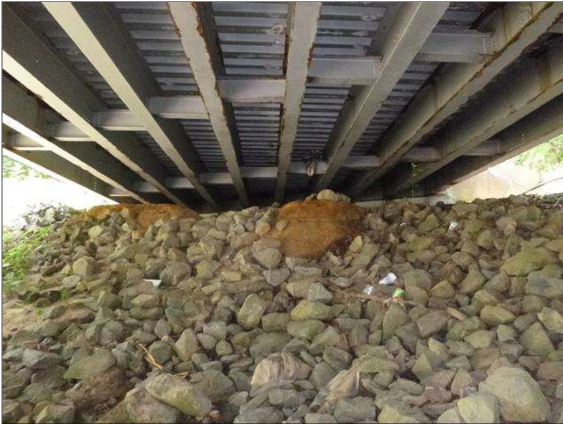
ABUTMENT 1, LOOKING SOUTH
