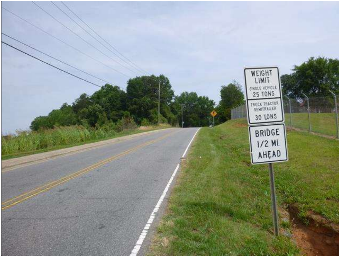
APPROXIMATELY 1/2 MILE SOUTH OF ABUT MENT 1, ADVANCE WARNING POSTING
